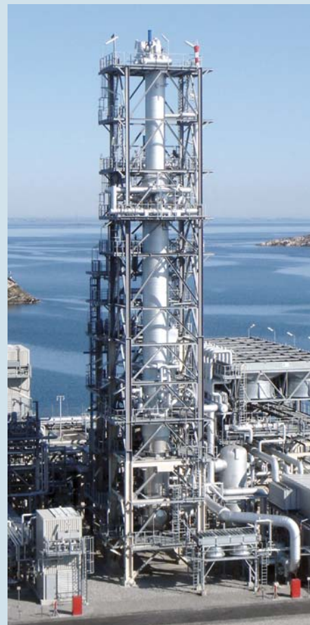
Fig. 3: Coil-wound heat exchanger (CWHE) at Stavanger LNG plant
