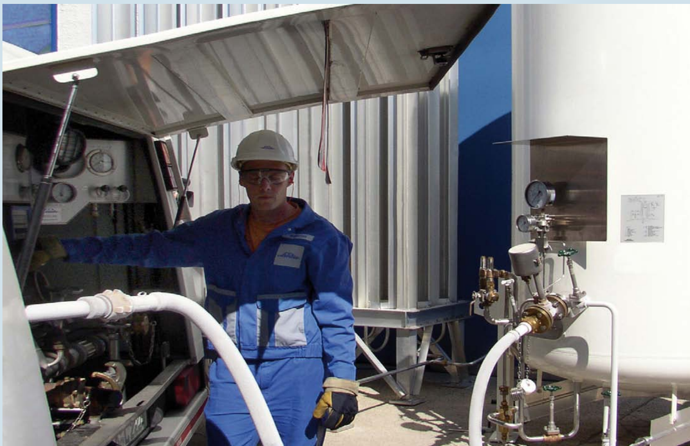
Truck unloading at LNG satellite station
