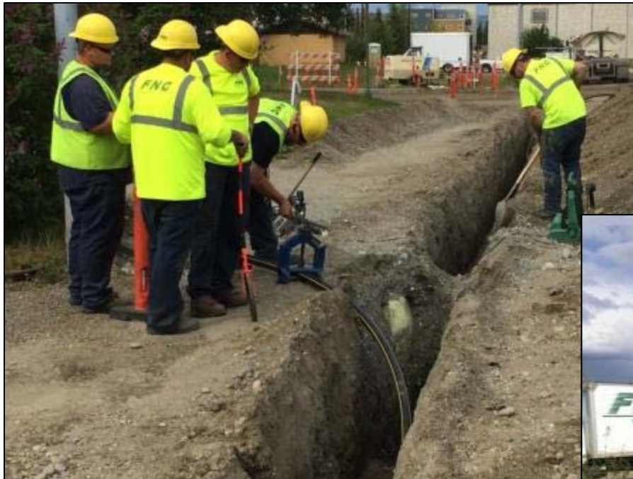
← Distribution pipe pressure testing
