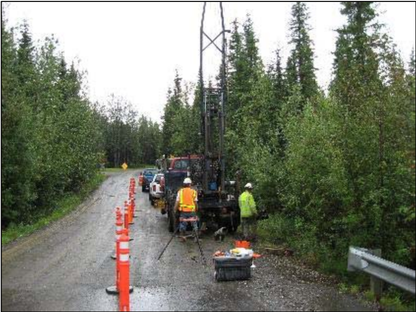
ROW core drilling
