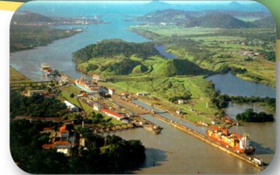
Panama Canal Expansion Project – Panama
