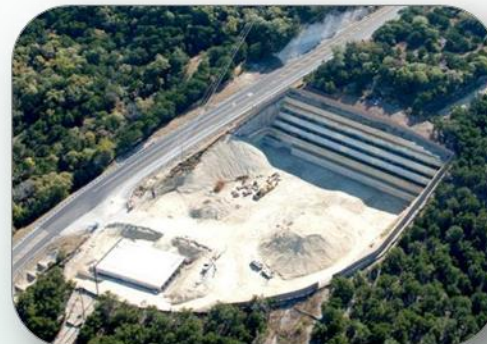
Austin Water Treatment Plant – Austin, Texas
