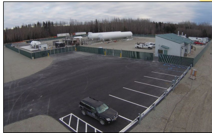
North Pole Storage & Vaporization
